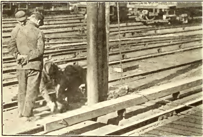
THIRD-RAIL TEMPORARILY PROTECTED BY WOODEN TROUGH
